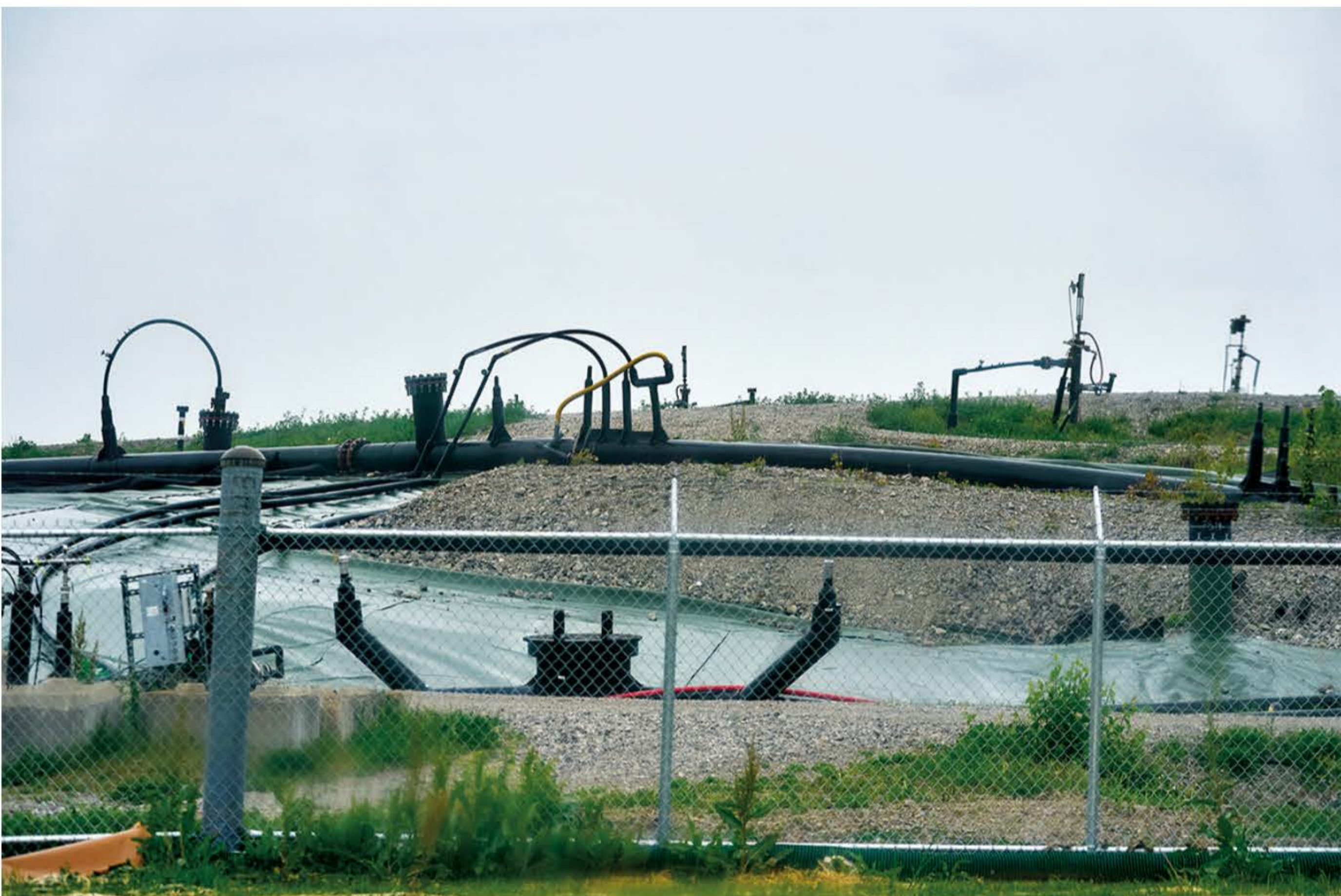
Gas extraction wells help limit the odor emanating from the Bridgeton Landfill. The facility, which is adjacent to the radiologically-contaminated West Lake Landfill, is experiencing a subsurface smoldering event, a chemical reaction that creates heat like a fire but lacks oxygen (Theo Welling/Riverfront Times).
